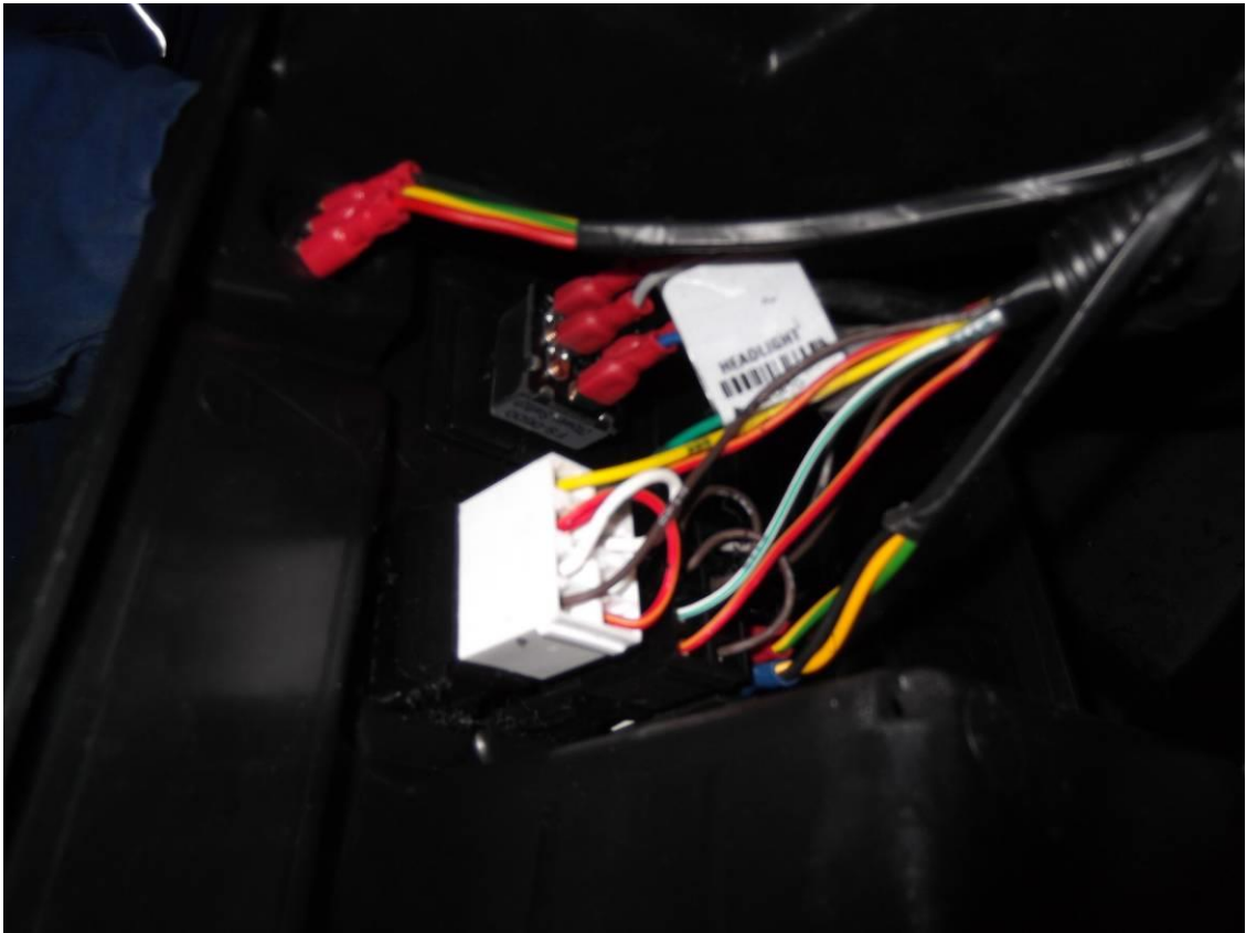
Inner view onto connected switches.
