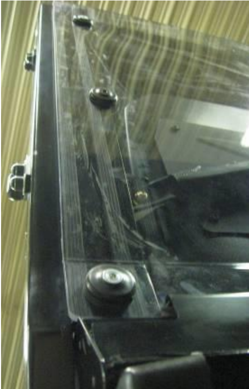
Rear panel after fixing – external view:
