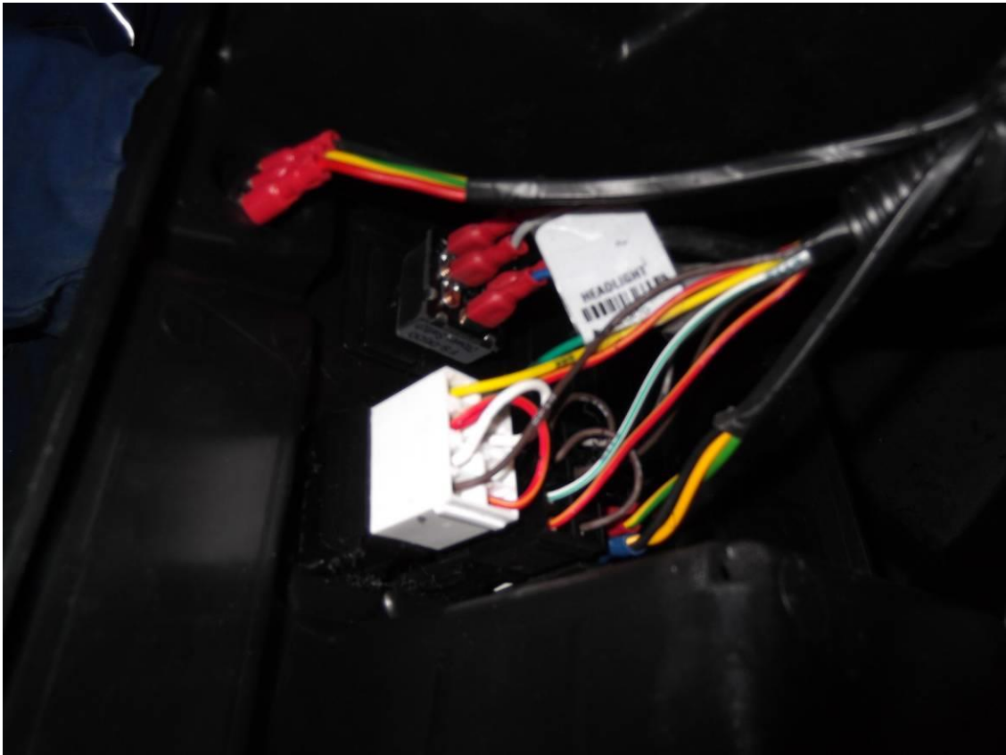
Inner view onto connected switches.
